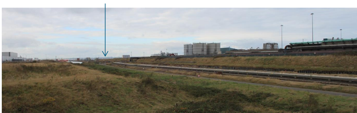
Figure 5-17 Viewpoint 17, Tees Dock Road, Day Time View
