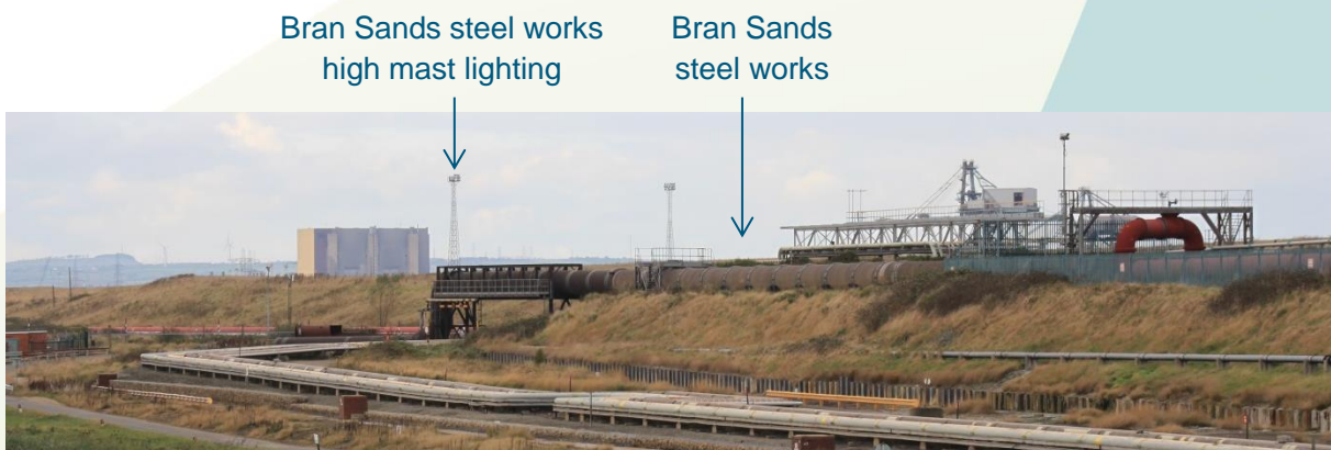
Figure 3-2 Existing high mast lighting within Bran Sands steel works
