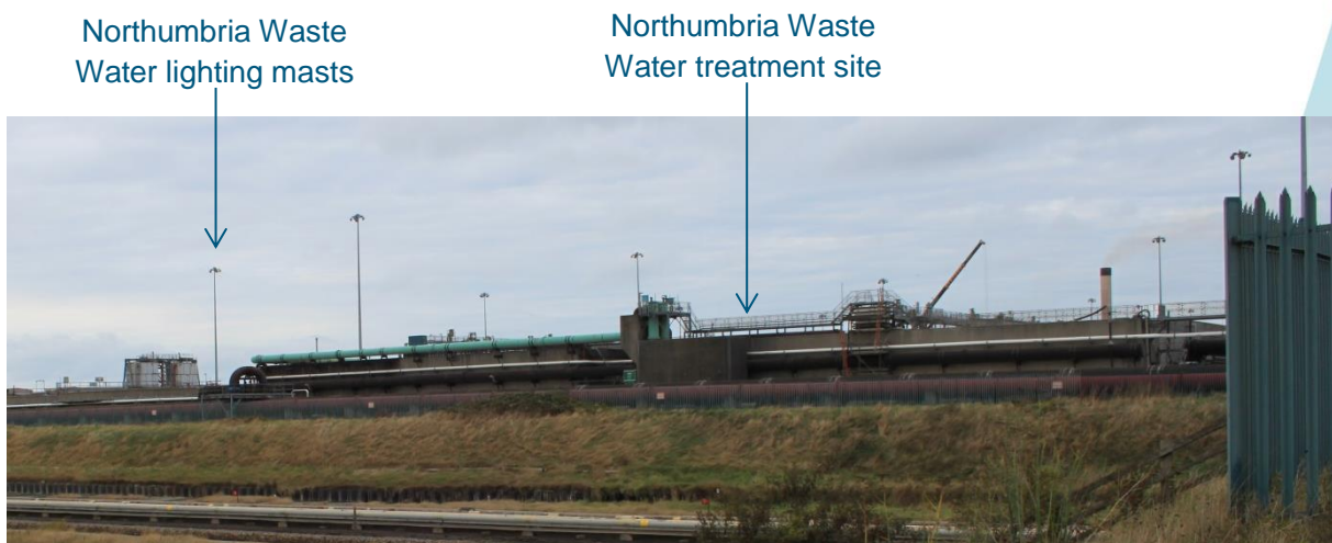
Figure 3-3 Northumbria Waste Water treatment plant high mast lighting
